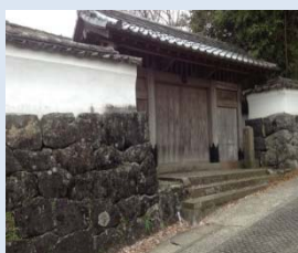
Roofed gate of the Hara House (Kashima-City)
