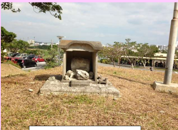
Façade of the small shrine
